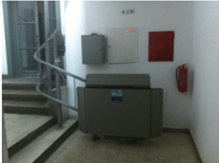
Figure 1.12: Second floor disabled elevator 1
