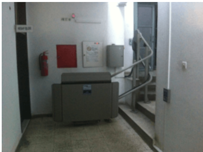
Figure 1.13: Second floor disabled elevator 2
